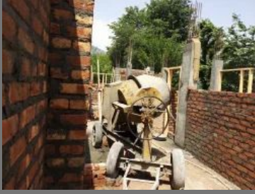
Building Construction Services For Hospital
