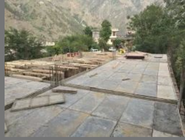
Building Construction Services For Mall
