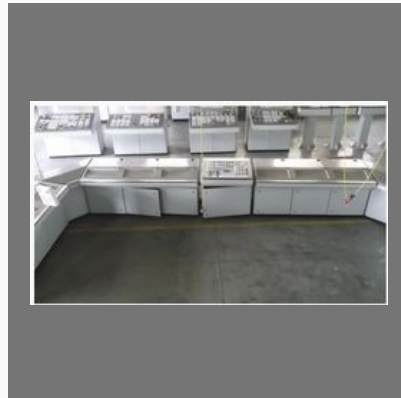
Low Maintenance Control Desk
