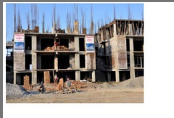
School Building Construction Services
