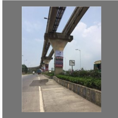
Monorail Boards Service
