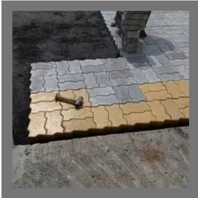
Paver Block Road Construction Service
