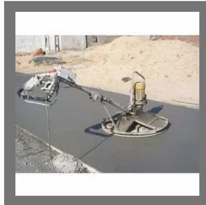
Water Bound Macadam RCC Road Construction Service
