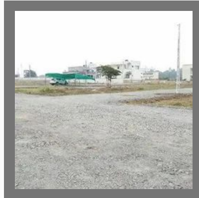
Concrete Road Construction Service
