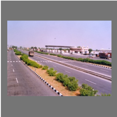
6 Way Highway Infrastructure Development
