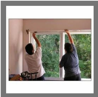
Aluminum Window Installation Service
