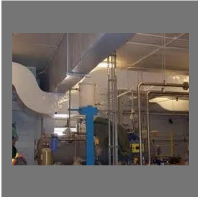
Duct Installation Service
