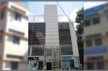
Commercial Building Construction Services
