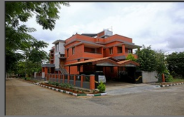
Industrial Building Construction Services
