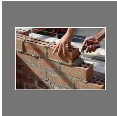
Civil Construction Contractor
