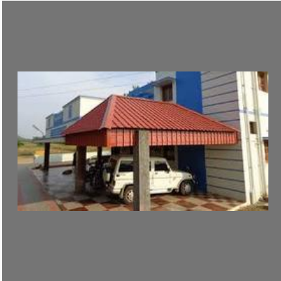
Roofing Fabrication Work
