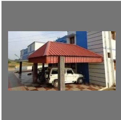
Roofing Fabrication Work
