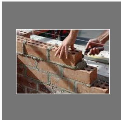
Civil Construction Contractor
