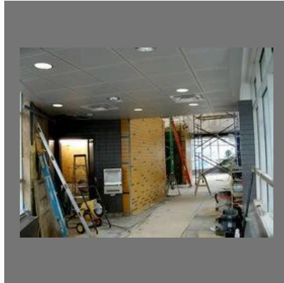
Civil Work Service
