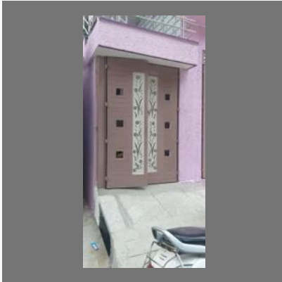
Automatic Entrance Gate
