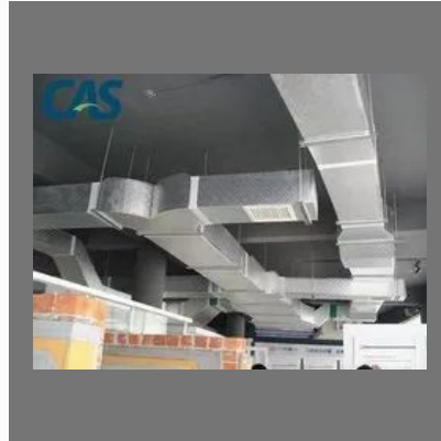
GI Duct Fabrication Work
