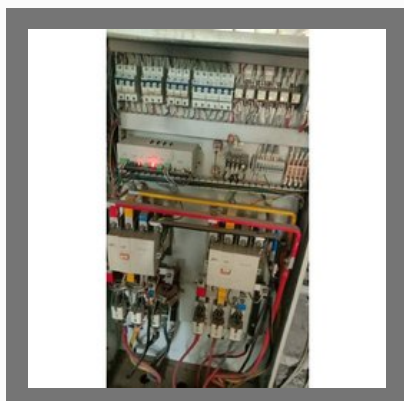
AMF Control Panel Repair Service
