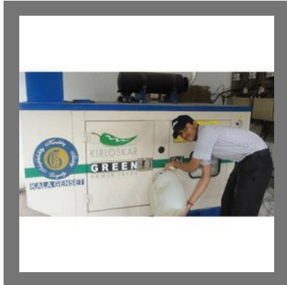
Generator Maintenance Services
