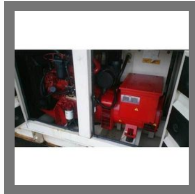
Heavy Generator Maintenance Service
