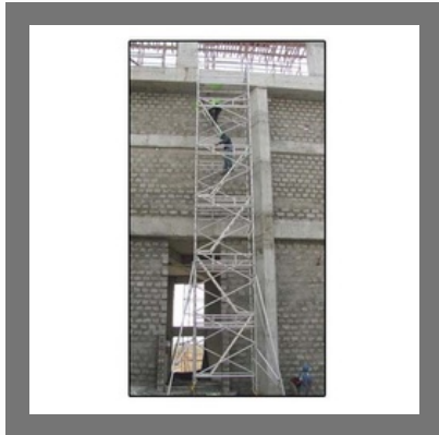
Construction Scaffolding Systems
