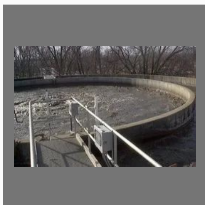
industrial waste water treatment plant
