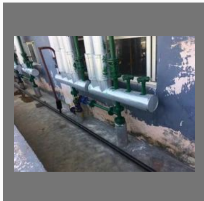
Industrial Piping System
