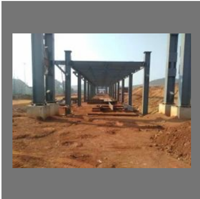
Pipe Bridge Fabrication Service
