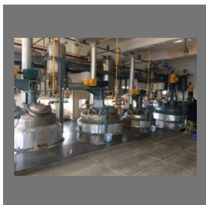
Ss Pipeline Works
