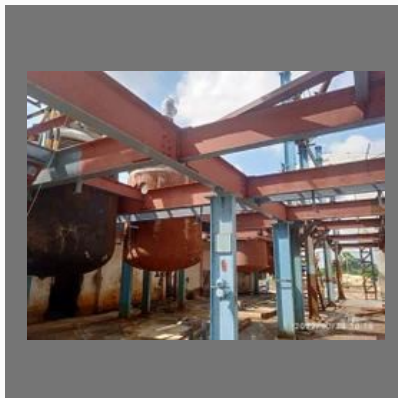
Heavy Structural Erection Works
