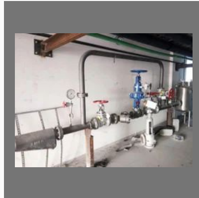
CI Pipe Line Fabrication Services
