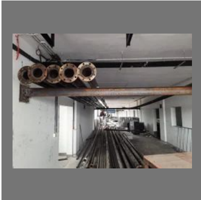
CS/MS Piping Fabrication Service
