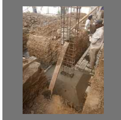
School Building Construction Services
