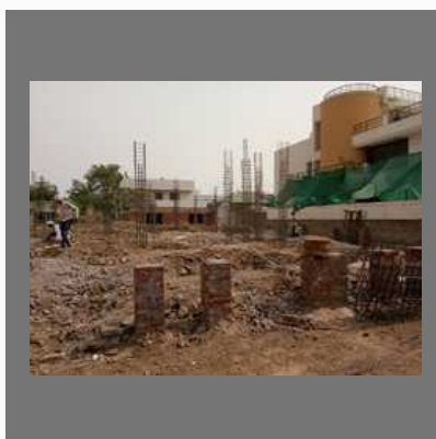
House Construction Services
