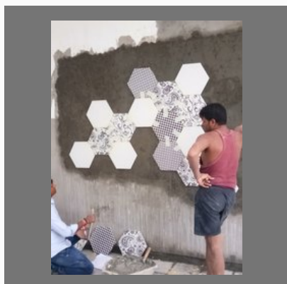
House Construction Services
