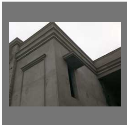
House Construction Services
