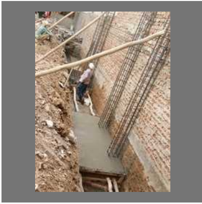
House Construction Services
