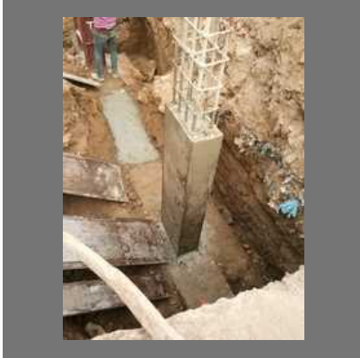
School Building Construction Services
