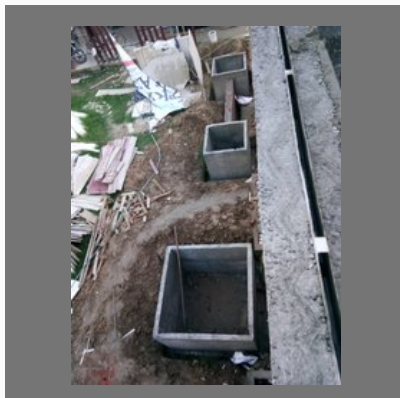
House Construction Services
