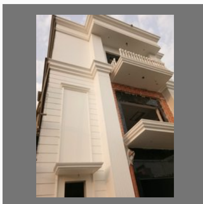
House Construction Services
