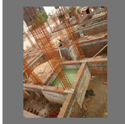
House Construction Services
