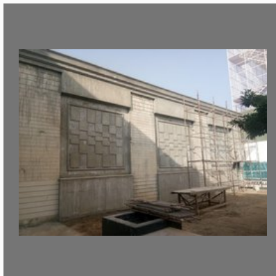
House Construction Services
