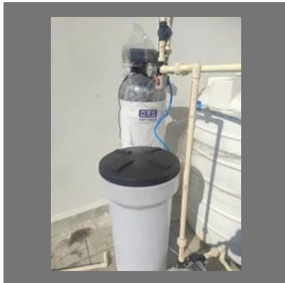
ORG Automatic Water Softener
