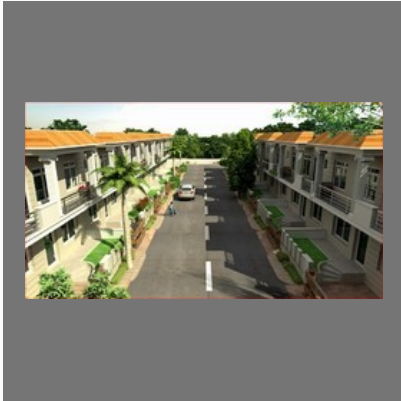
4BHK Flats Construction Services
