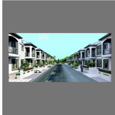
Luxury Villas Construction Service
