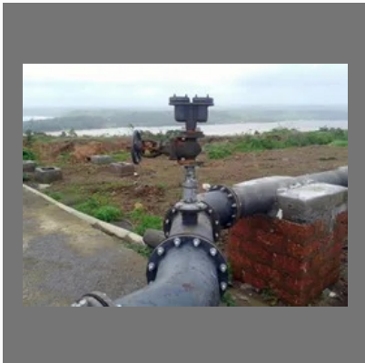
DI Pipeline Services
