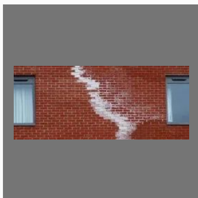
Salt Efflorescence
