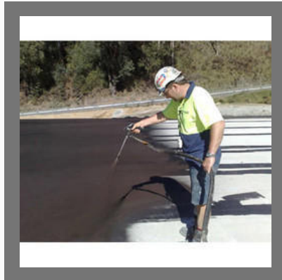
Liquid Membrane Waterproofing Service
