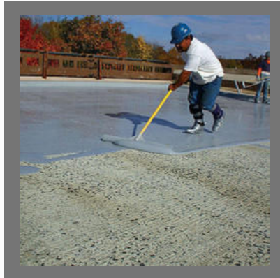
Terrace Waterproofing Service
