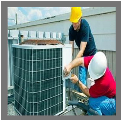
Air Conditioning Maintenance Services
