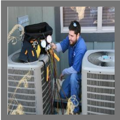
HVAC Installation Services
