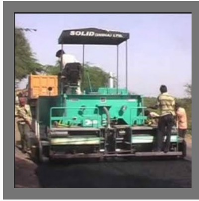
Road Construction Services
