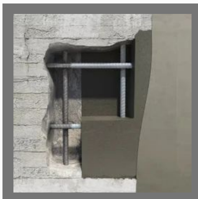
Concrete Repairing & Maintenance
