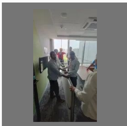
Building Glass Replacement
