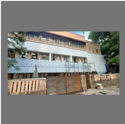
Aluminum ACP Cladding Service
