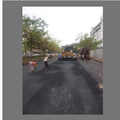
BT Roads Construction Services
