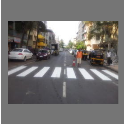
Road Construction Services
