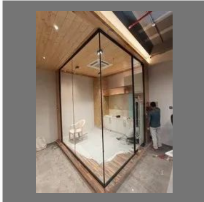
Glass Office Enclosure
