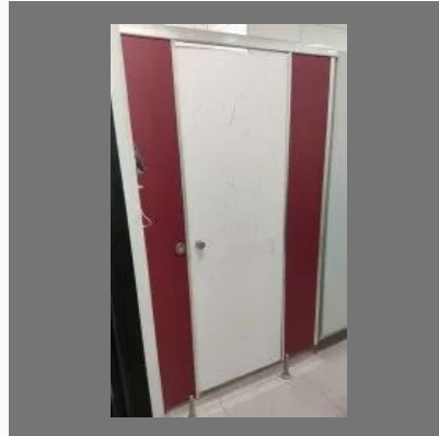
Office Toilet Cubicle
