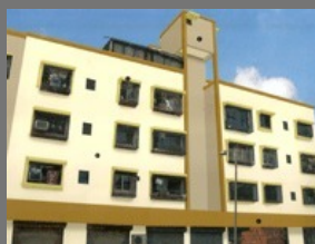
Building Repairs & Painting Service
