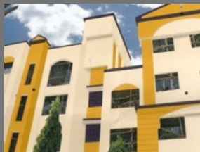
Structural Repair Service
