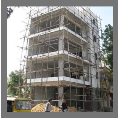
School Building Construction
