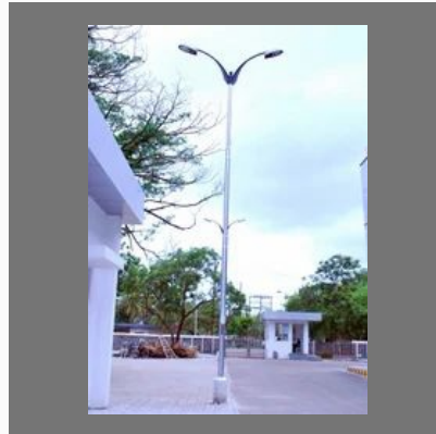
Installation Of Street Light Turnkey Electrical
