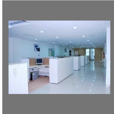
Installation Of Light Fittings Turnkey Electrical
