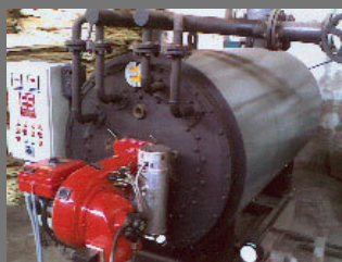
Thermic Fluid Heaters
