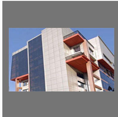
A.C.P Cladding & Structure
