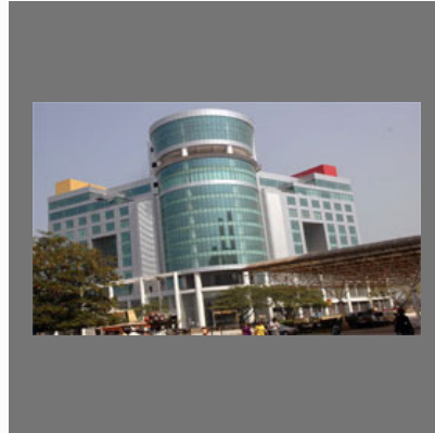
A.C.P Cladding & Structure
