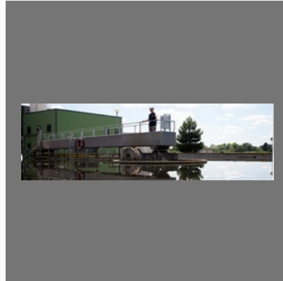
Storm Water Drain System
