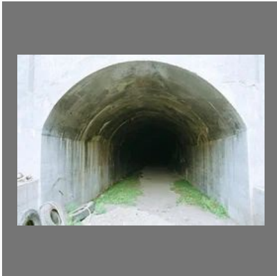
Tunnels Construction Services
