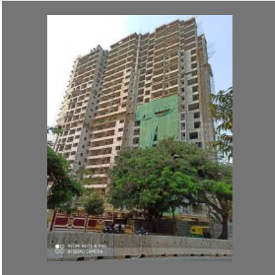
Commercial Building Construction Services
