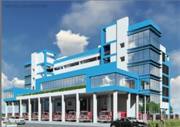
Five Pump Fire Station Project
