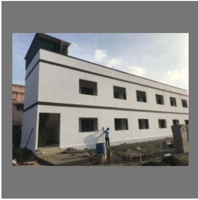
School Building Construction
