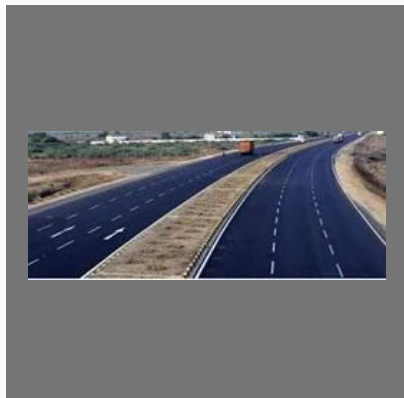
Road Runways And Elevated Corridors Services
