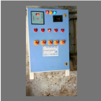
Automatic Power Factor Panel
