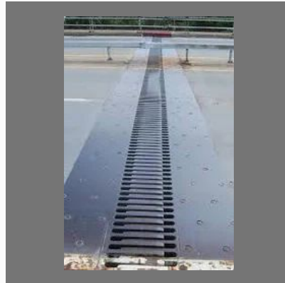
Bridge Expansion Joint
