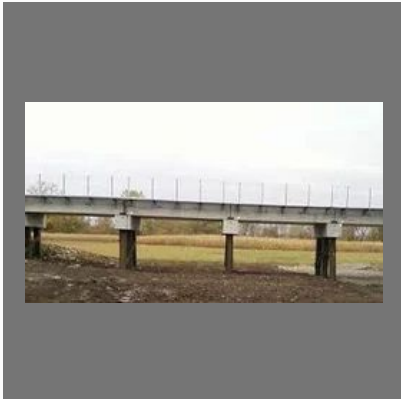
Bridge Repairing Service
