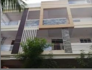
House Building Construction Service
