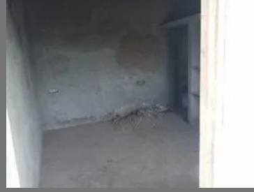
House Building Construction Service
