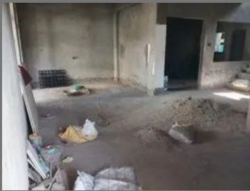
House Building Construction Service
