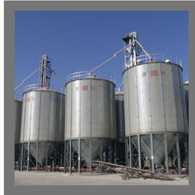
Cement Storage Silo
