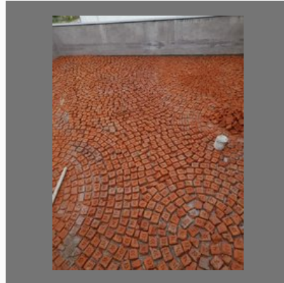
Brick Bat Coba Terrace Waterproofing
