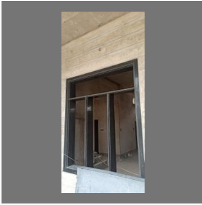
Grenite Fitting Contractor Ji
