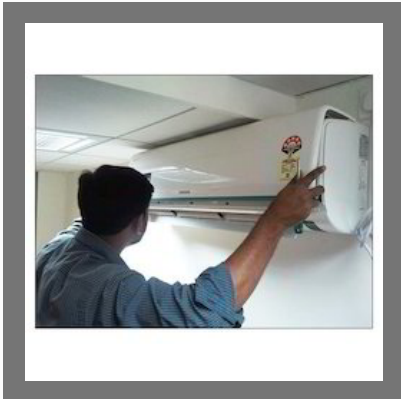
Split AC Repairing Service
