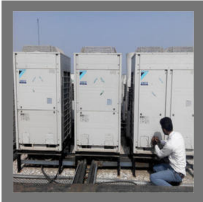
VRF System Repairing Service
