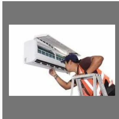
Panasonic Air Conditioner Repairing Service
