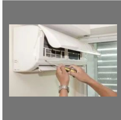
Haier Air Conditioner Repairing Service
