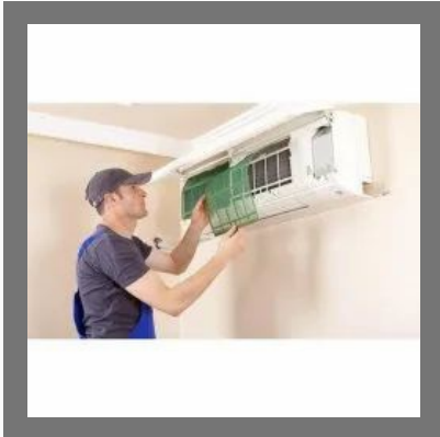
Panasonic Air Conditioner Repairing Service
