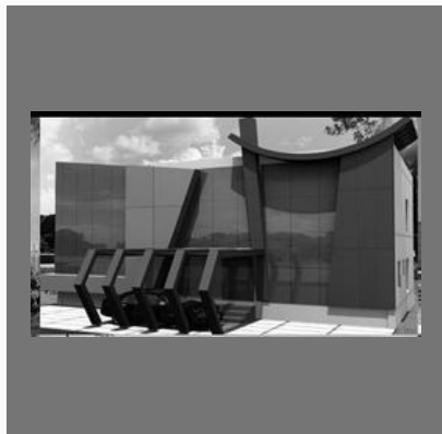
Corporate Office Building Services
