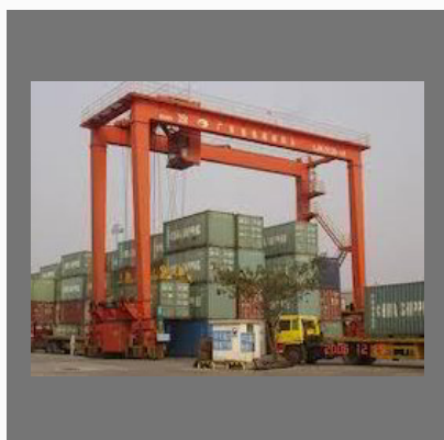
Container Handling Crane Service
