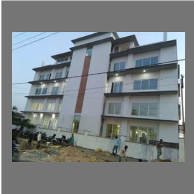
Hostel Interior Service
