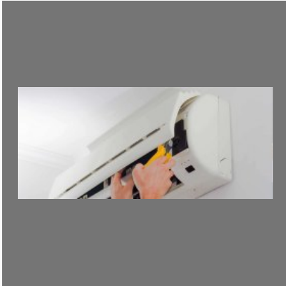
Split Air Conditioner Installation Service
