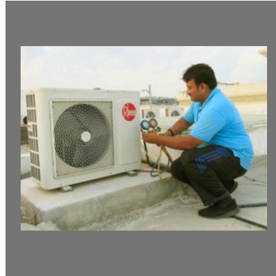
Air Conditioner Repairing
