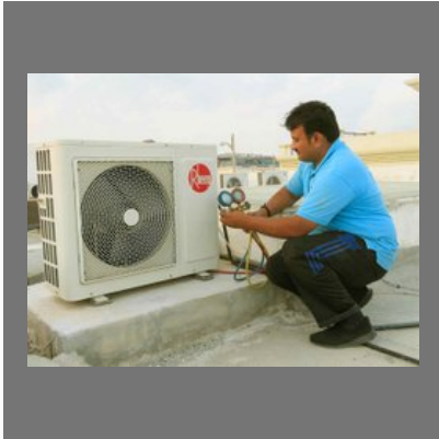
Ac Repairing Services
