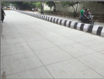
Cement Concrete Road Construction Servic...
