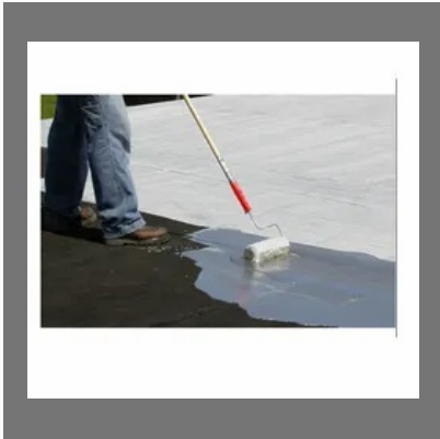
School Building Waterproofing Services
