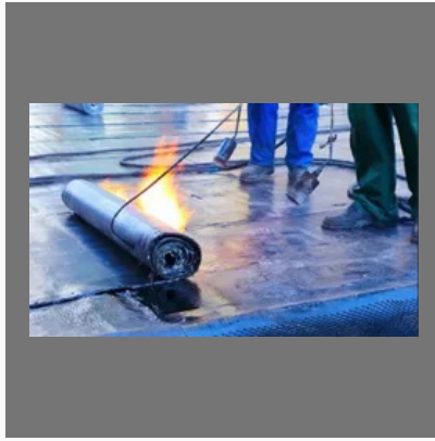
Commercial Building Waterproofing Services
